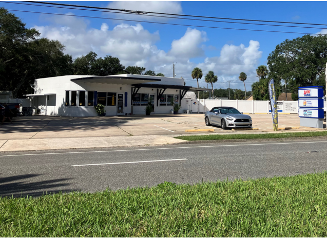
CRA Small-Scale CFPI Grantee: JARS Holding New Smyrna, Inc. 646 N Dixie Fwy- After Improvements (2021)
