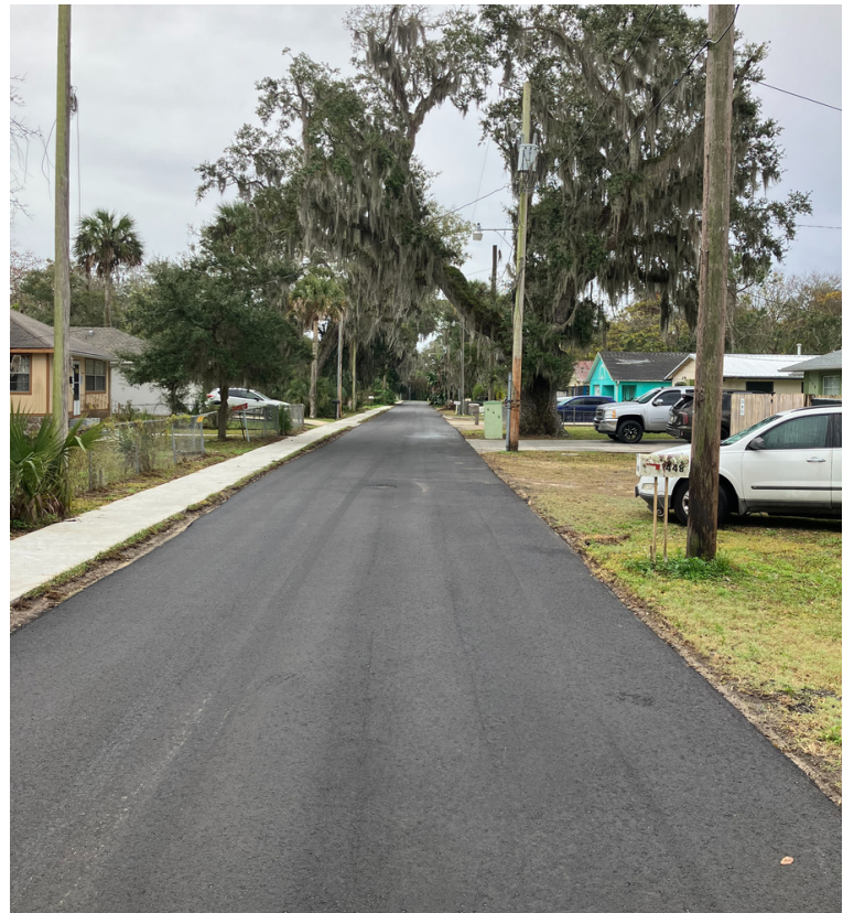
Palm Street Project as February 16, 2024 looking south
