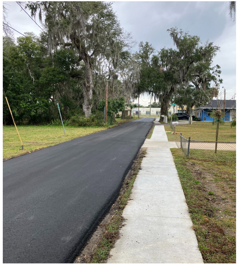
Palm Street Project as February 16, 2024 looking north
