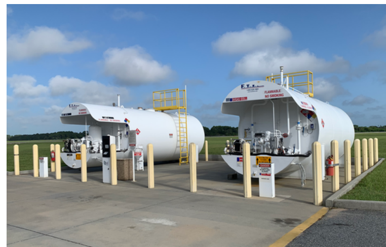
Existing Fuel Farm Facilities at NSB Municipal Airport
